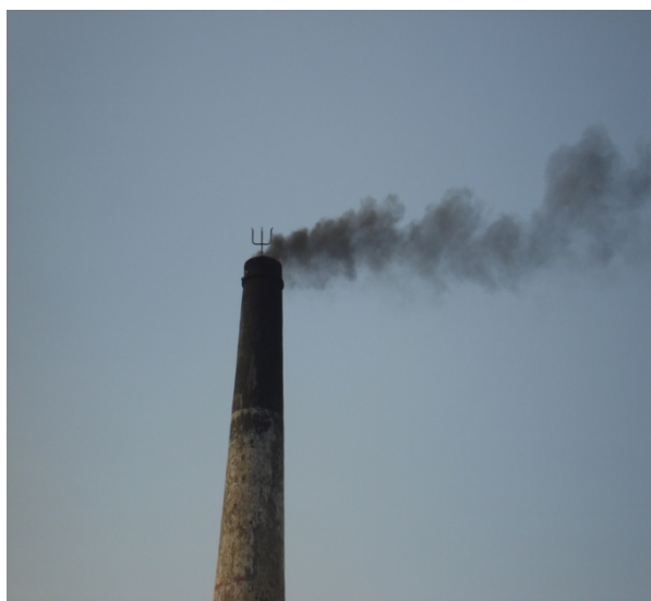
Black smoke from a FCBTK during fuel charging
