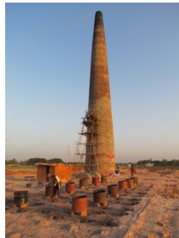
Photo showing longer coal feeding zone
