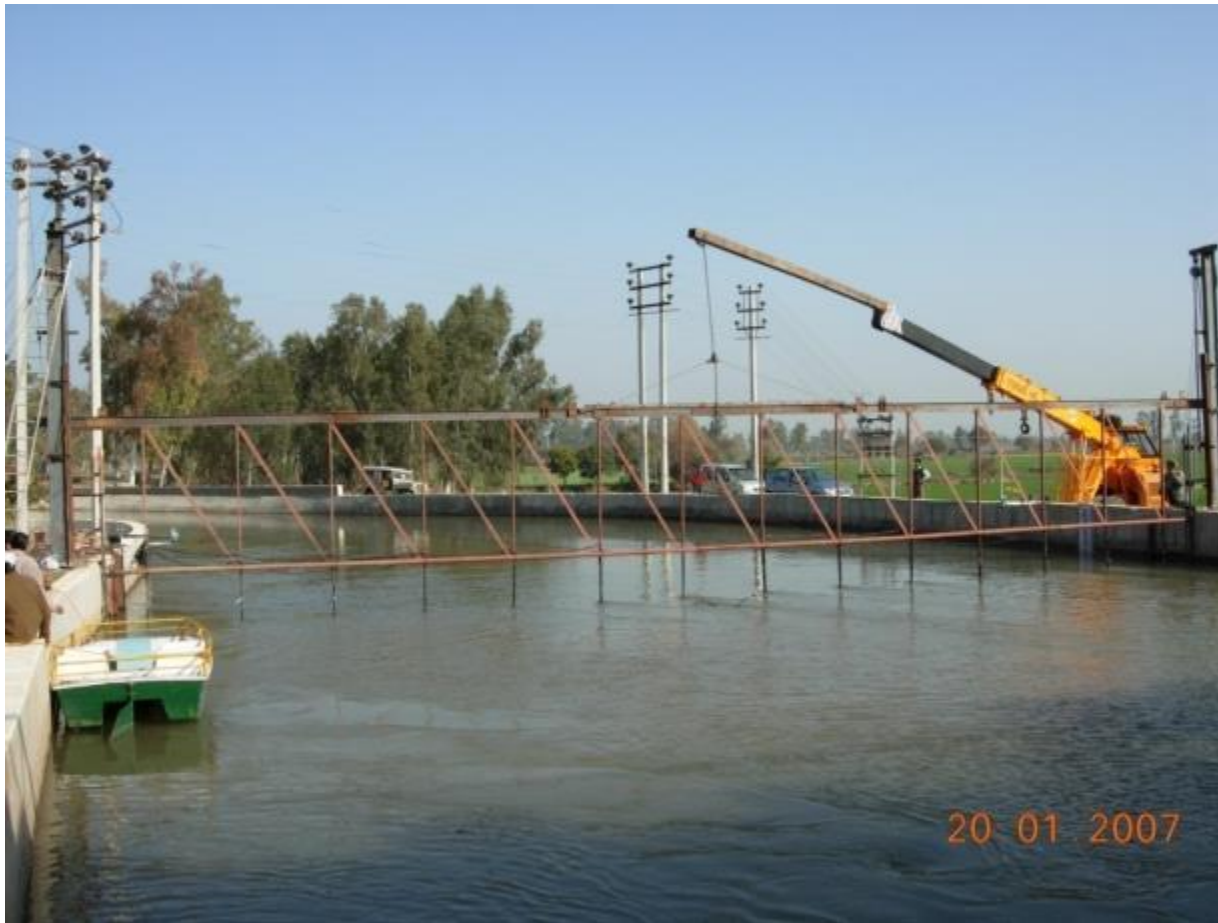
(b) Frame Lowered
