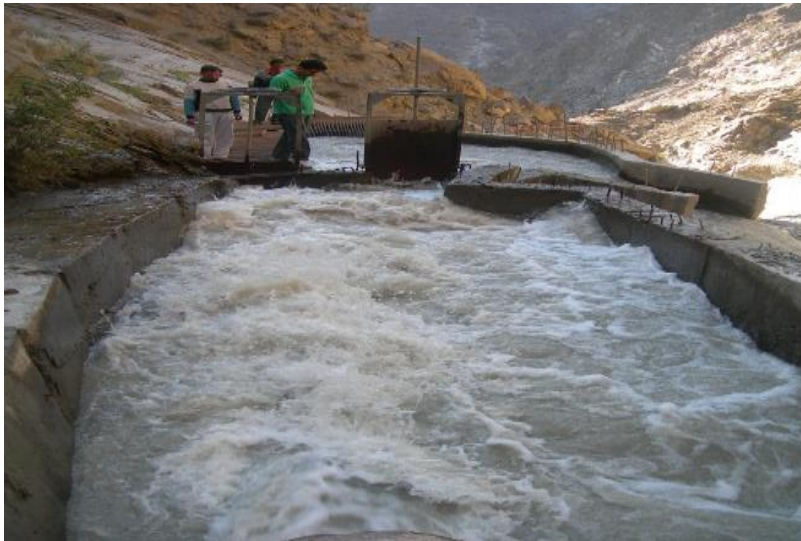
BEFORE FLASH FLOOD
