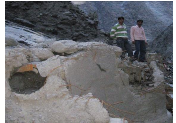
AFTER FLASH FLOOD
