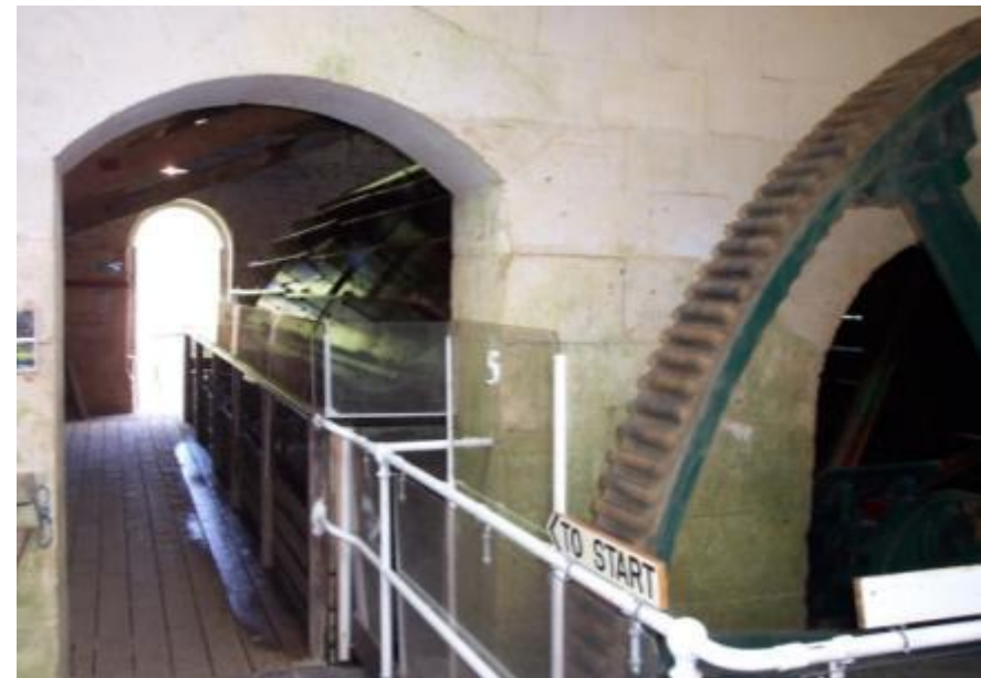
Calverton Water-Pumping station, UK
