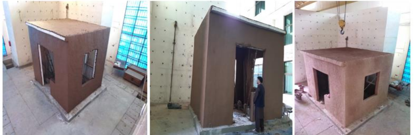
SMIP plaster finishing and curing
