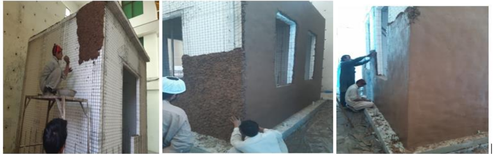
SuperMud plastering with steel smoother on panels.
