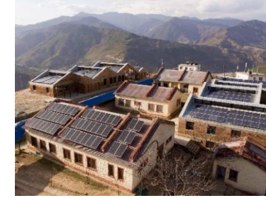
Hospital: 100 kWp Hospital Ac coupled Solar PV System
