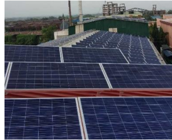
Pharmaceuticals: 117 kWp On-Grid System with net metering
