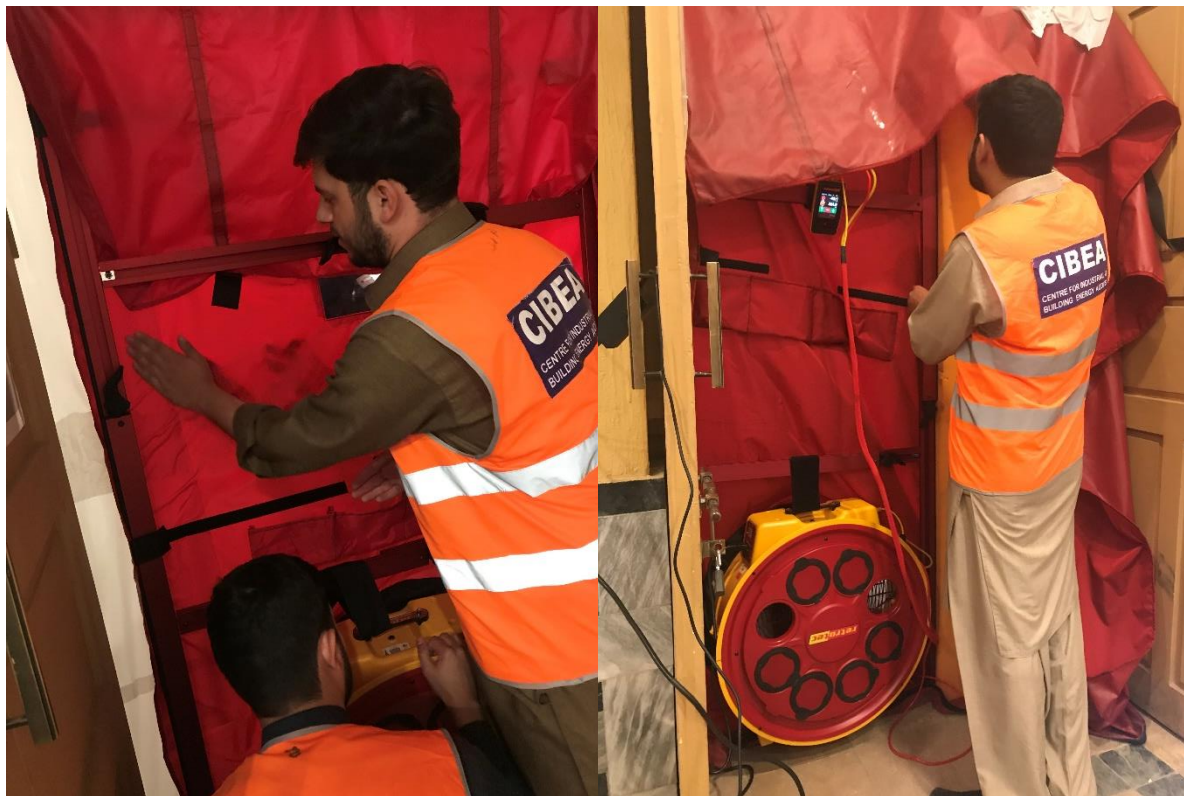
Team CIBEA setting the blowerdoor equipment
