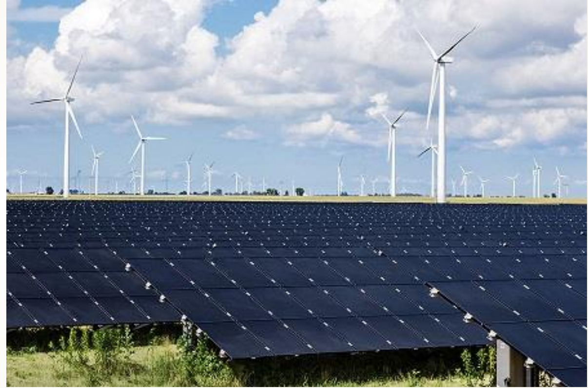
Solar and Wind Farm 12-18 months to build
