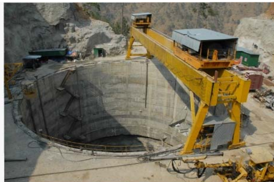
Surge Shaft (PHPA-II)
