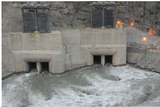
Diversion Tunnel- Inlet end ( PHPA-I)
