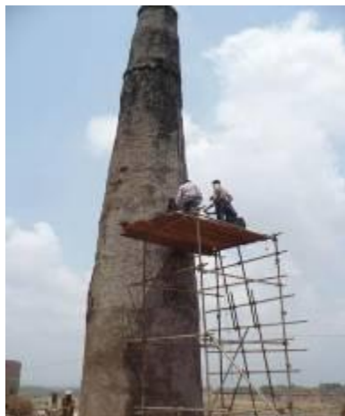
Photo: EPA monitoring stack emissions
