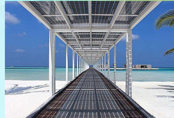
960 kWp Solar PV installation at Finolhu Villas Resort
