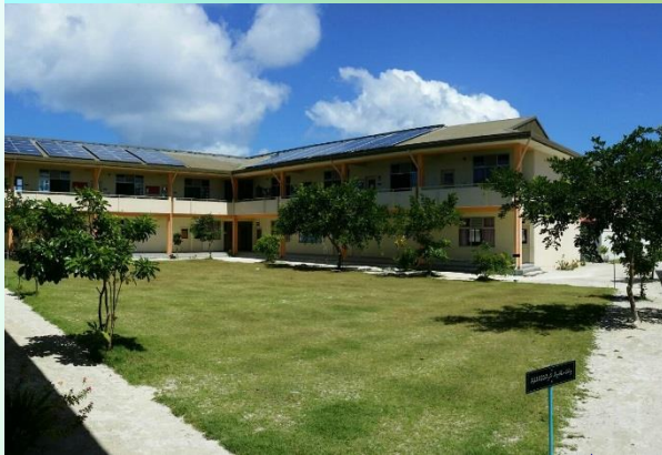
558 kWp solar PV in 3 public buildings in Gdh. Thinadhoo
