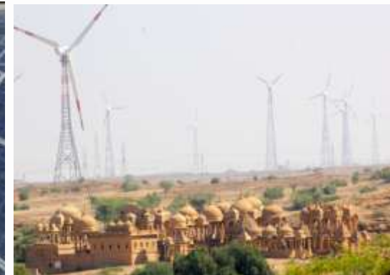
Wind Farm in Jaisalmer, Rajasthan India
