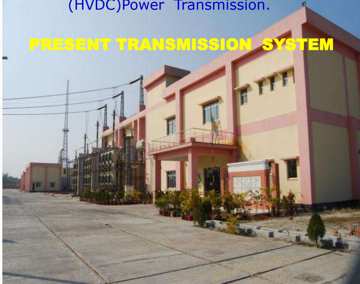
Control Building of HVDC Station, Bangladesh
